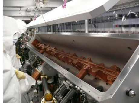
Figure 3: ReA RFQ during the final installation
